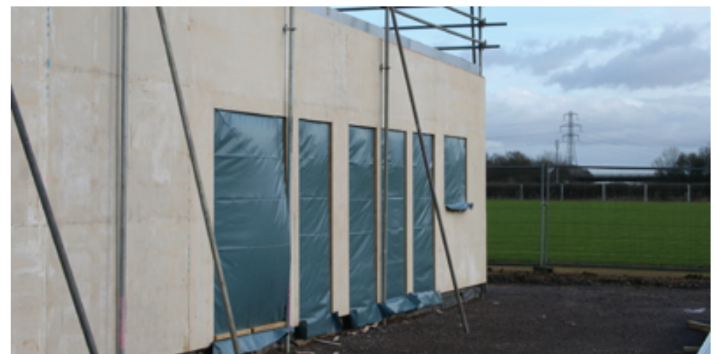
CONSTRUCTION OF NEW CLUBHOUSE JANUARY 2015
