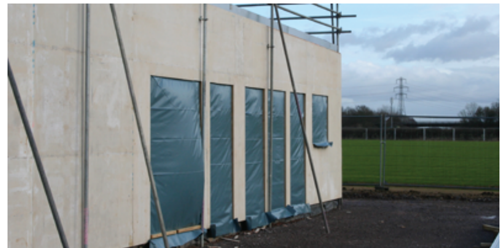
CONSTRUCTION OF NEW CLUBHOUSE JANUARY 2015
