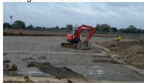
Footings for the Clubhouse....
